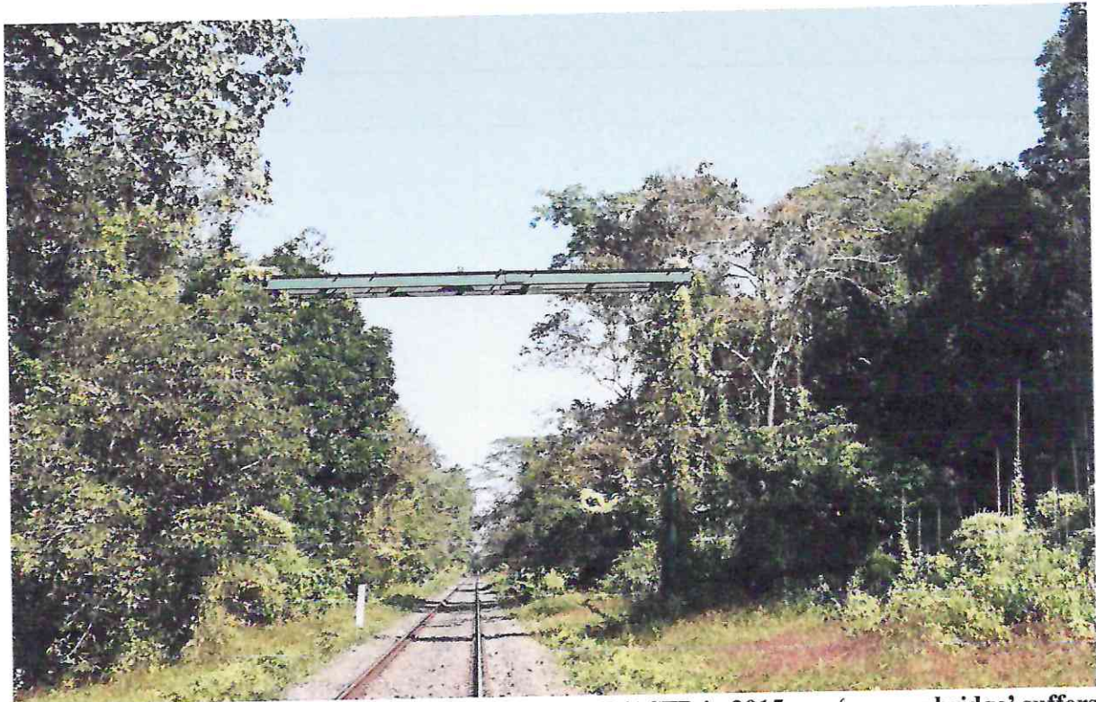
Figure 3: The iron structure constructed by the NEFR/ASFD in 2015 as a ‘canopy bridge’ suffers from several design flaws vis-à-vis the target species Hoolock gibbon’s preferred mode of locomotion (brachiation) and habits making it unusable for them
